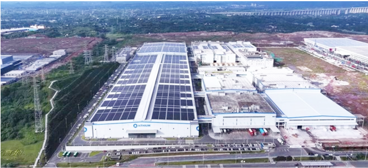
Hithium Chongqing Base
