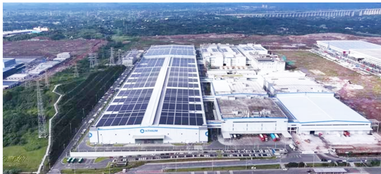
Hithium Chongqing Base
