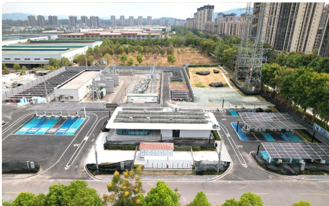
Chongqing, China 400kW solar, 2*860kWh ESS, 12*160kW charging station
